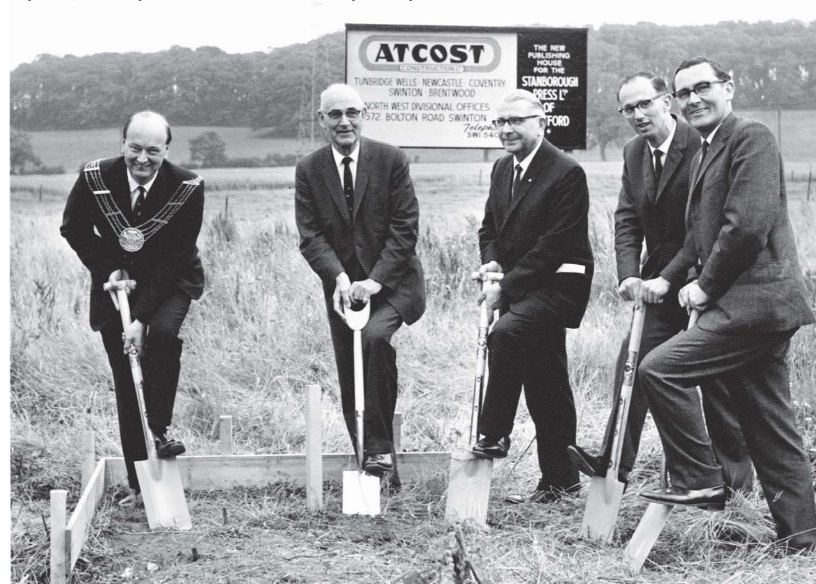
In August of 1965, a contract was signed with Atcost Construction Ltd. to build a new Stanborough Press building in Grantham
